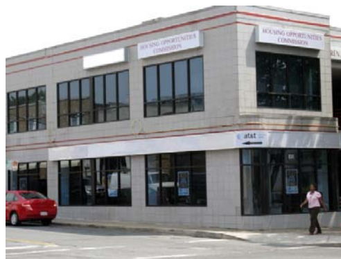
Silver Spring HOC Customer Service Center
